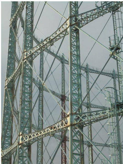
Granton No 1 Gasholder at the start of the refurbishment, and the bell to contain gas that has now been removed. © Mark Watson, HES
