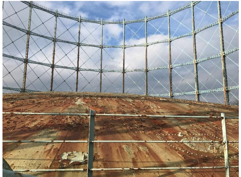
Granton No 1 Gasholder at the start of the refurbishment, and the bell to contain gas that has now been removed. © Mark Watson, HES
