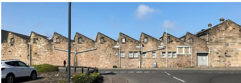
The Glasgow (and Lancashire) style of weaving shed: steeply angled north lights, overhead shafting and narrow spans, at Peter Grieg's Victoria Linen Works in Kirkcaldy, Fife. (photos @ Mark Watson)
