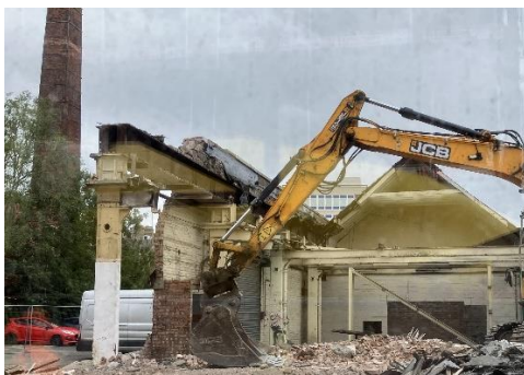
Dudhope Works, Dundee, chimney and weaving shed, built in 1837: equal-sided spans lit north and south. Steel girders installed below line shaft brackets to enable installation of beams into looms. An extension had been added in 1893- the pillars and girders on the left. Is/ was this the oldest surviving power loom weaving shed in Scotland? Photo © Mark Watson, HES
