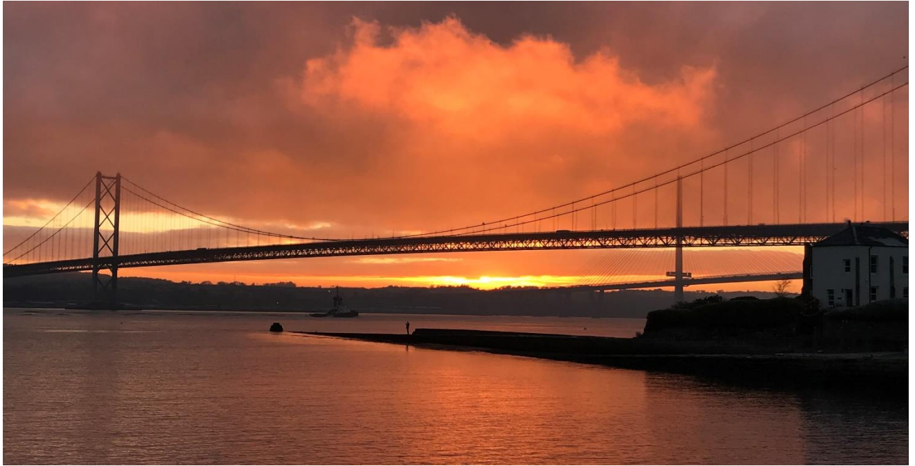
The Forth Road Bridge. Photo © Mark Watson, HES
