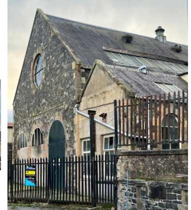
Dudhope Works, Dundee, chimney and weaving shed, built in 1837: equal-sided spans lit north and south. Steel girders installed below line shaft brackets to enable installation of beams into looms. An extension had been added in 1893- the pillars and girders on the left. Is/ was this the oldest surviving power loom weaving shed in Scotland? Photo © Mark Watson, HES
