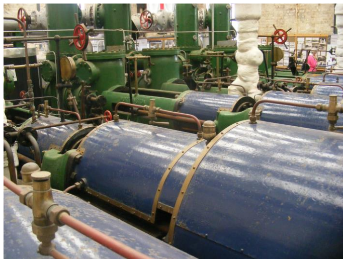
Fuel pumps, Lyness, Hoy
